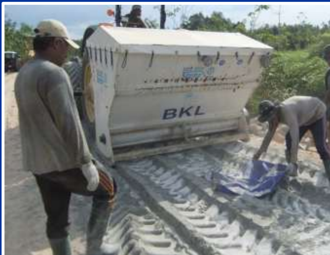
Spreading of NovoCrete®
