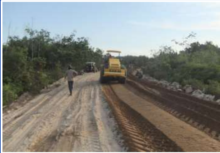
Static and dynamic compaction
