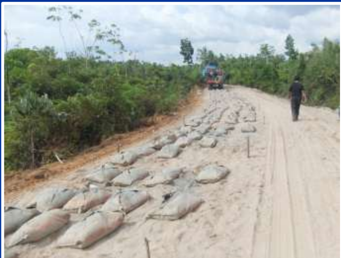
Manual distribution/spreading of cement
