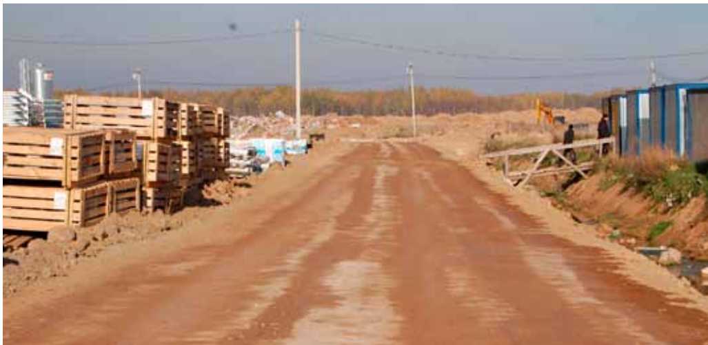
Area one day after compaction
