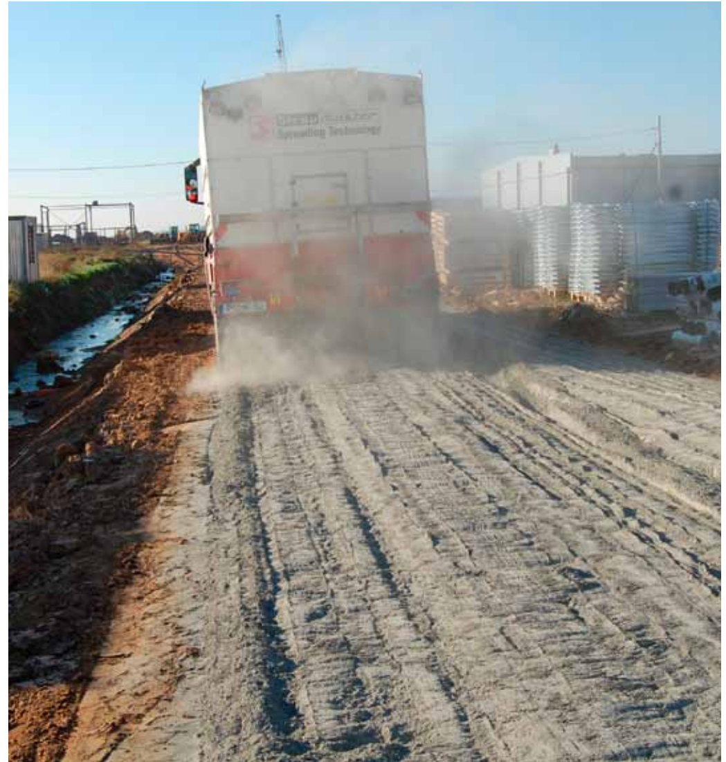
Spreading of cement
