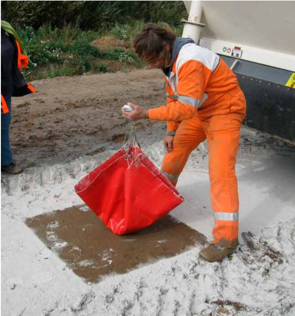
Check of the spreaded amount of NovoCrete®
