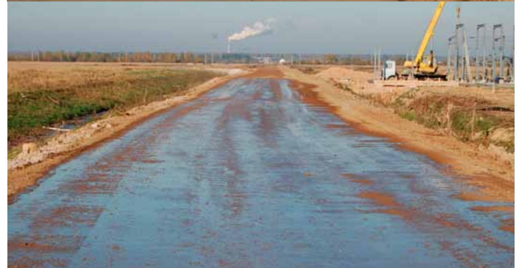
Irrigation as protection against evaporation
