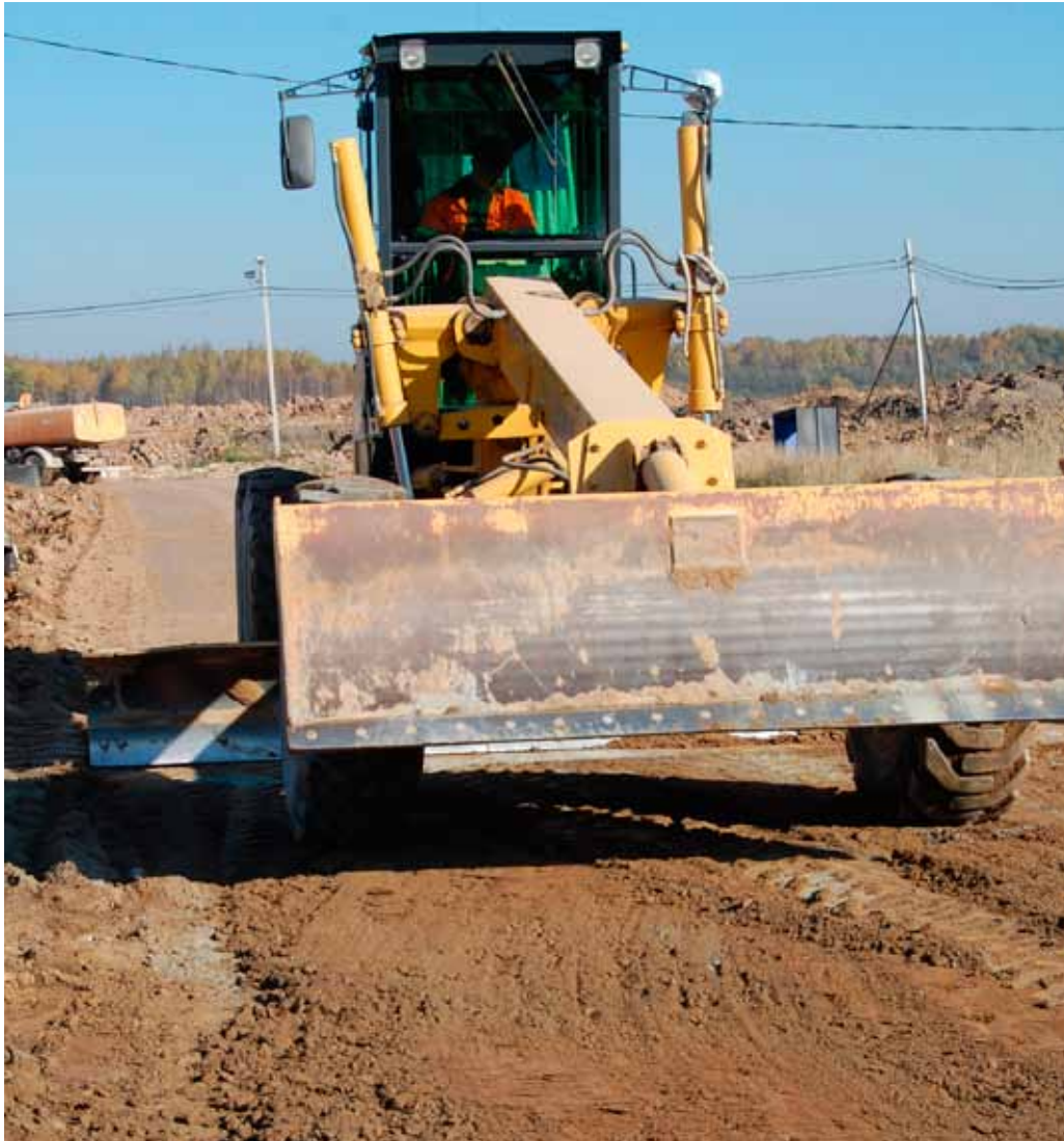
Use of the Grader for the levelling
