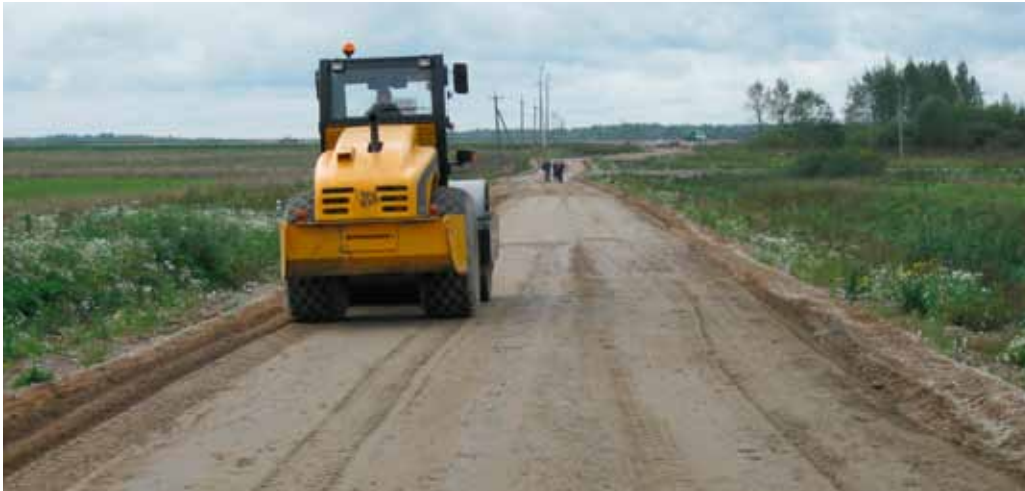
The steel drum roller was used for compaction
