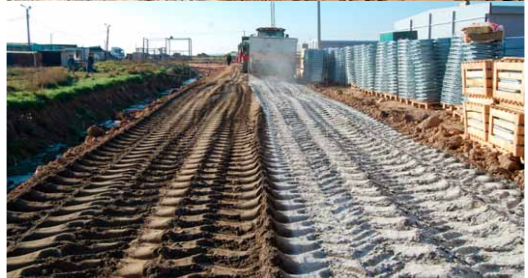
Spreading of the cement additive NovoCrete®
