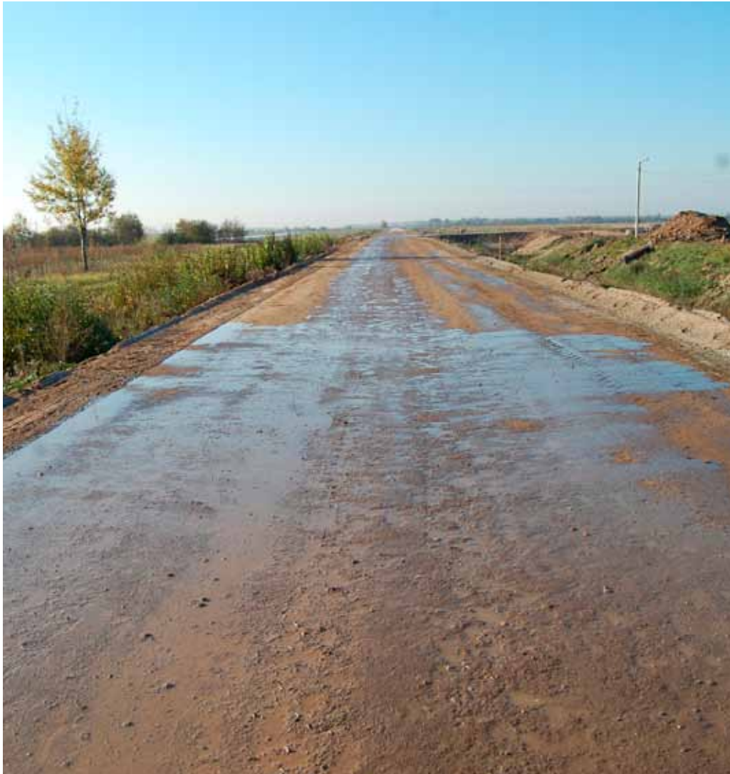
Area in the crossing section of gravel road and soils consisting of clay/silt after irrigation
