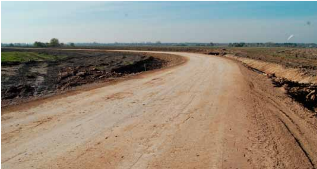
Finished section with soils consisting out of clay and silt
