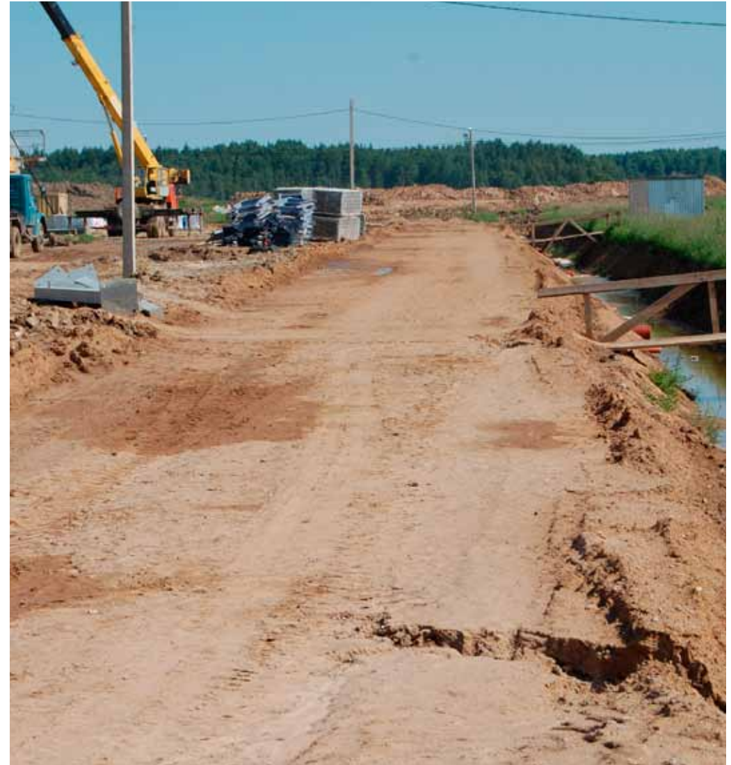
Initial situation before filling up the silty clay material
