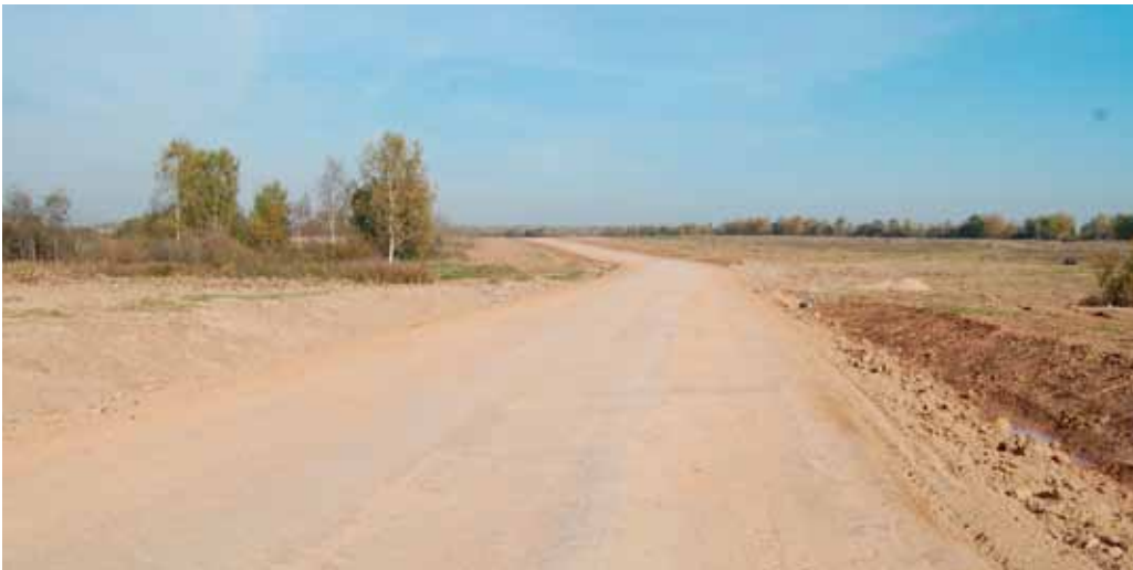
Finished section with soils consisting out of clay and silt
