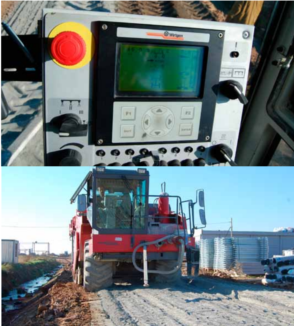
Milling of the binding agent material up to a milling depth of 0,45 m
