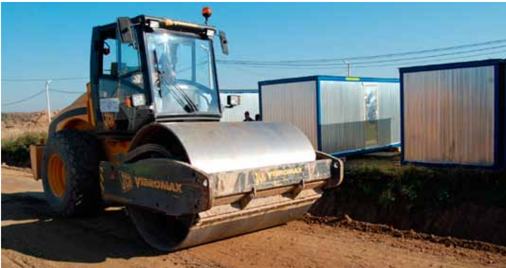
Dynamic and static compaction with steel drum roller (weight of 12 tons)
