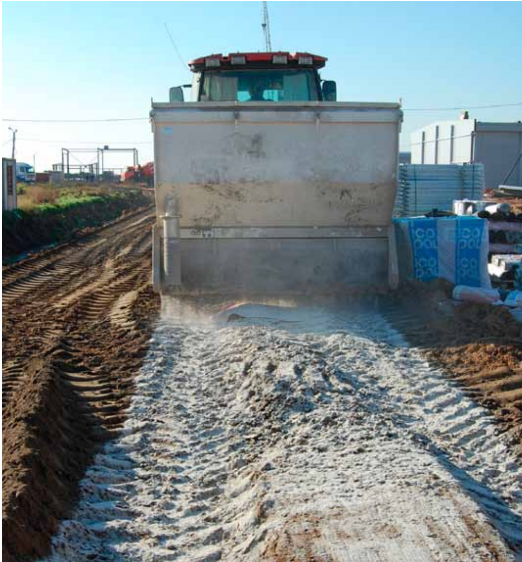
Tractor with attached spreader unit for the cement additive NovoCrete®
