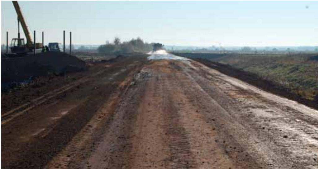
Permanent irrigation of the area
