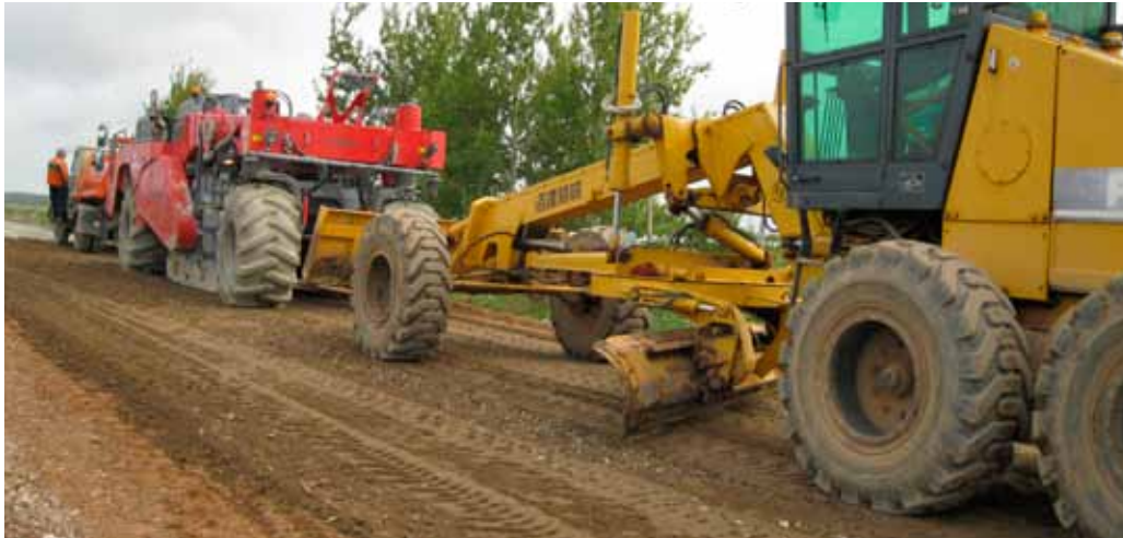
Use of a Grader for the levelling
