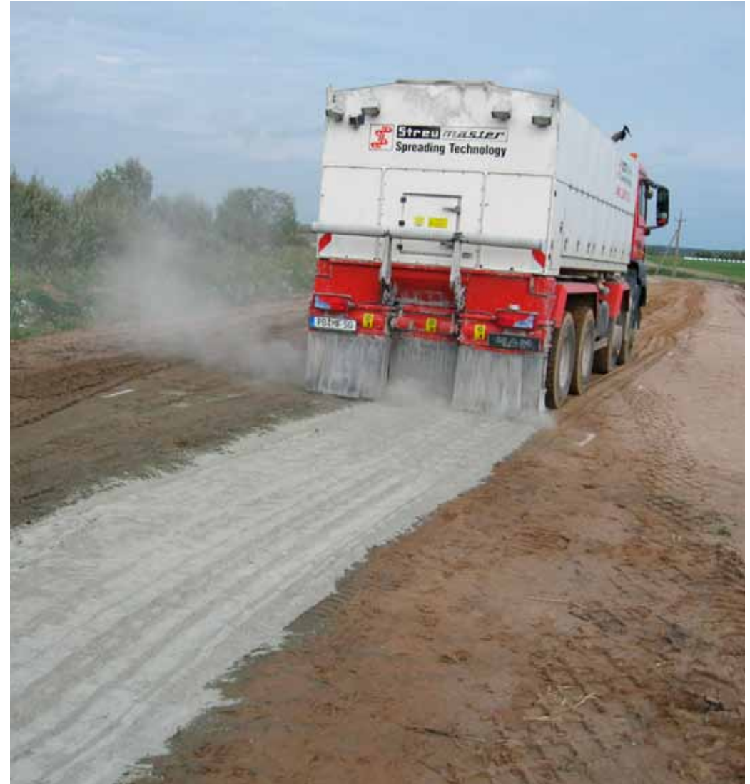
Spreading of the cement
