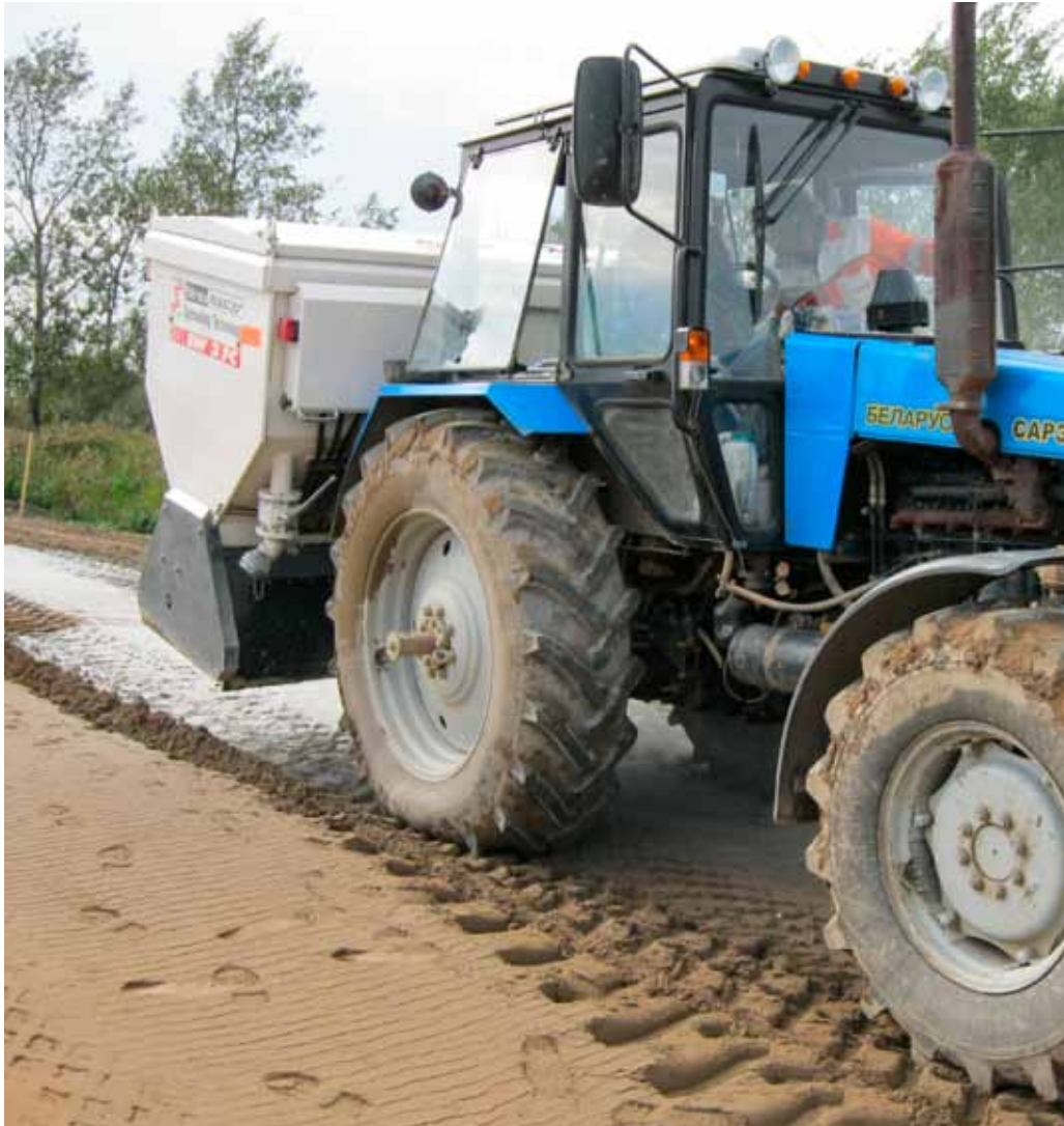
Tractor with the attached spreading unit for the cement additive NovoCrete®
