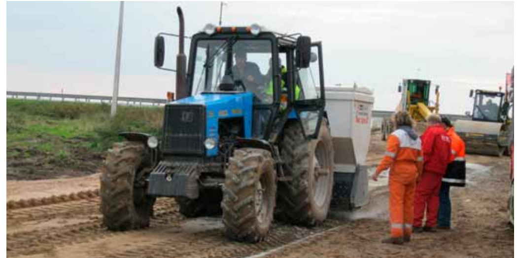
Spreading of the cement additive NovoCrete®
