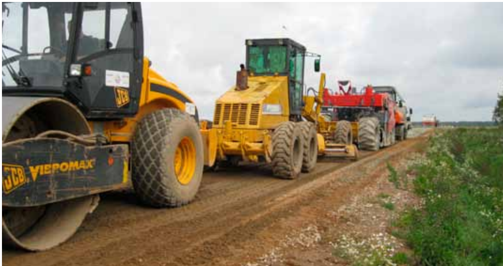
Spreader, milling machine, Grader and steel drum roller in action
