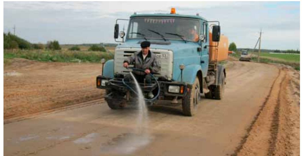
Irrigation of the surface
