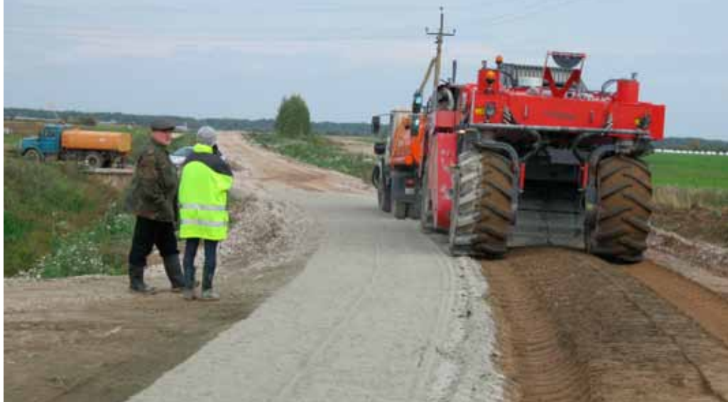
Milling of the binding agent up to a milling depth of 0,45 m
