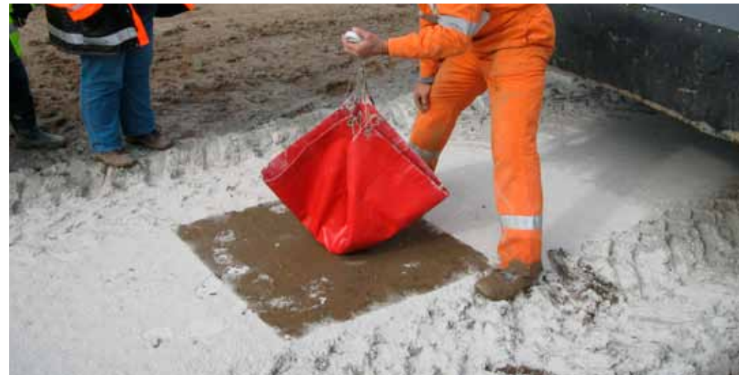
Checking of the spreaded amount of binding agent
