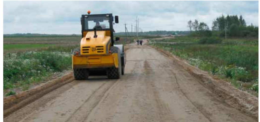
Static and dynamic compaction
