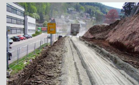
Spreading cement + NovoCrete
