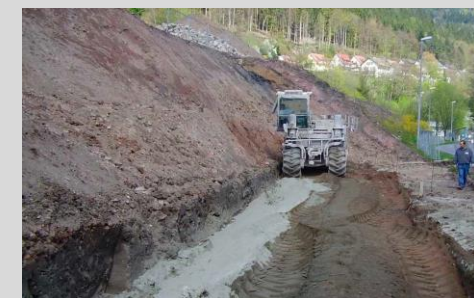
Milling of cement + NovoCrete
