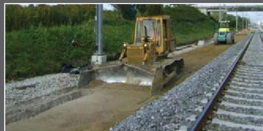
Leveling the Surface
