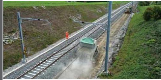
Spreading the NovoCrete® - Cement Mixture
