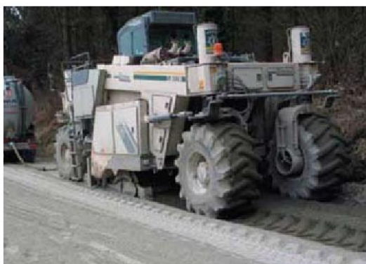
5 Mixing of NovoCrete®, cement and water with a soil-mixing Machine
