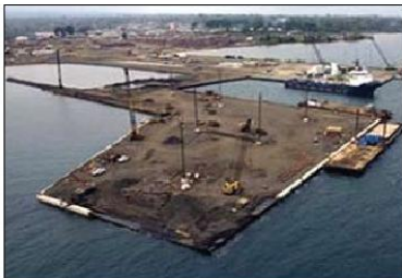
Equatorial Guinea, Malabo Harbor premises: Making the base layer of the pier on which the container traffic is performed with NovoCrete® Surface: 40,000m 2 Date: 2002-2003 Time needed: 4 weeks Mixture: 50 kg/m 2 (98% cement + 2% NovoCrete) Milling Depth: 30 cm
