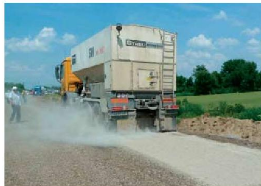
4 Spreading of NovoCrete® and cement mixture with spreading machine
