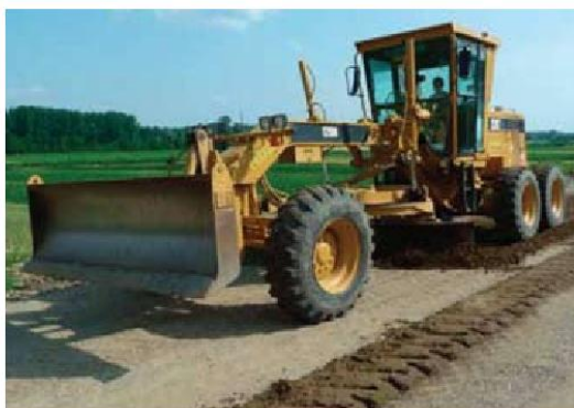
3 Leveling with a grader
