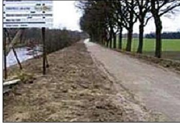
Gemert-Bakel, Holland Bicycle paths: Making the base and frost preventing layer with NovoCrete® of the areas used by the cyclists. Using the nature dential surface without adding any asphalt layer. Surface: 22,000m Date: August 2006 Time needed: 1 week Mixture: 170 kg/m 3 Milling Depth: 25 cm
