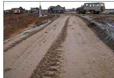
Russia, Kaluga VW production building: Making the NovoCrate® and frost preventing layers of the production building Surface: 10,000m 2 Date: October 2006 Time needed: 1 week Mixture: 52 kg/m 2 (98% cement + 2% NovoCrete) Milling Depth: 40 cm
