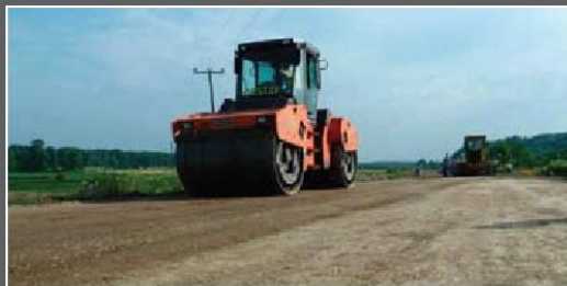
Making the Static and Dynamic compression with Steel Drum Roller
