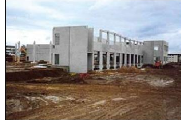
Germany, Ostfildern-Scharnhausen Shipping company: Making the base and frost preventing layer of the building, plant ground and transportation roads of a shipping company. Surface: 10,000m Date: December 2000 Time needed: 2 weeks Mixture: 150 kg/m 3 Milling Depth: 100cm (in three stages)
