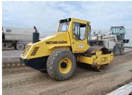
8 Leveling the surface with single drum roller
