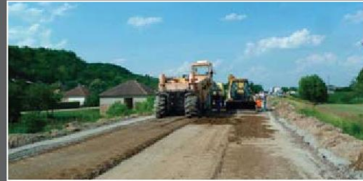
Mixing the NovoCrete®- Cement-Soil-Old Asphalt Layer by adding water
