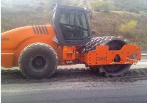
7 Compaction the surface with vibrating drum roller
