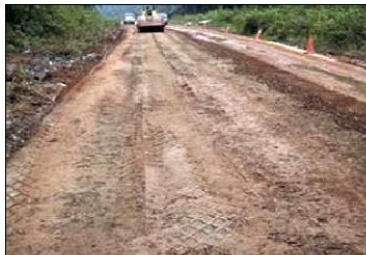
Malaysia, Jalan Pakoti Timur renewal of the agricultural Road: Renovating the agricultural road goes between palm plantations and used by heavy load vehicles with nature-identical surfaces Surface: 11 km Date: August 2006 Time needed: 6 weeks Mixture: 60 kg/m 2 (98% cement + 2% NovoCrete) Milling Depth: 30 cm
