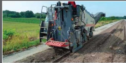
Crushing the old asphalt layer
