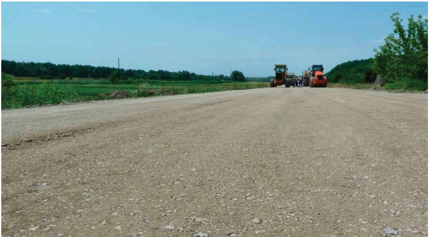
9 Result: Base mechanic is finished and it is ready for spreading the bitumen-asphalt layer
