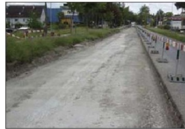
Rheinfelden, Switzerland Strengthen K292 state highway: Making the base and frost preventing layer with NovoCrete® for strengthen the state highway. Surface: 990m Date: May 2006 Time needed: 2 days Mixture: 180 kg/m 3 Milling Depth: 30 cm
