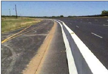
USA, Daimler Chrysler Laredo Texas test lane: Renewal of a lane and making NovoCrete® base layer Surface: 10,000m 2 Date: May 2004 Time needed: 2 weeks Mixture: 60 kg/m 2 (98% cement + 2% NovoCrete) Milling Depth: 25 cm
