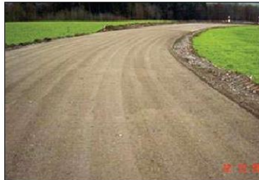
Switzerland, Unterlunkhofen state highway: Renewal of a lane and making NovoCrete® base layer Surface: 7,500m 2 Date: December 2006 Time needed: Crushing 2 days, road construction 4 weeks Mixture: 62 kg/m 2 (98% cement + 2% NovoCrete) Milling Depth: 25 cm
