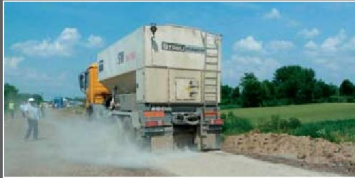
Spreading the NovoCrete®- Cement Mixture
