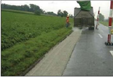
Alikon-Abtwil, Switzerland widening K38 state highway: Making the base and frost preventing layer with NovoCrete® for widening the state highway. Surface: 200m Date: August 2001 Time needed: 1 day Mixture: 180 kg/m 3 Milling Depth: up to 30 cm
