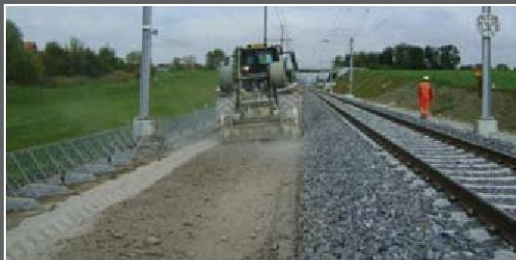
Milling the NovoCrete® - Cement Mixture
