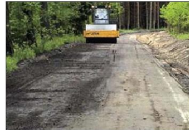
Poland, Renewal of the forest paths: Making the NovoCrate® base and frost preventing layers of the forest paths used for timber transportation Surface: 25,000m 2 Date: June 2004 Time needed: 2 weeks Mixture: 52 kg/m 2 (98% cement + 2% NovoCrete) Milling Depth: 25 cm
