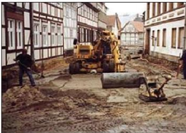
Salzwedel, Germany Construction of the sewage lines used by the "inter-plant mixing" processes: Making the base and frost preventing layer of the natural stone basins used for the "inter-plant mixing" Surface: 20,000m 2 Date: 2002-2003 Time needed: 4 days Mixture: 150 kg/m 3 Milling Depth: 30 cm
